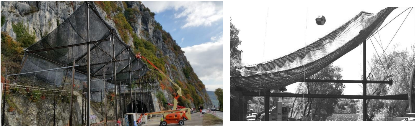
Figure 1: The temporary multi-layer rockfall gallery (left) and capture of the impact test (right)
