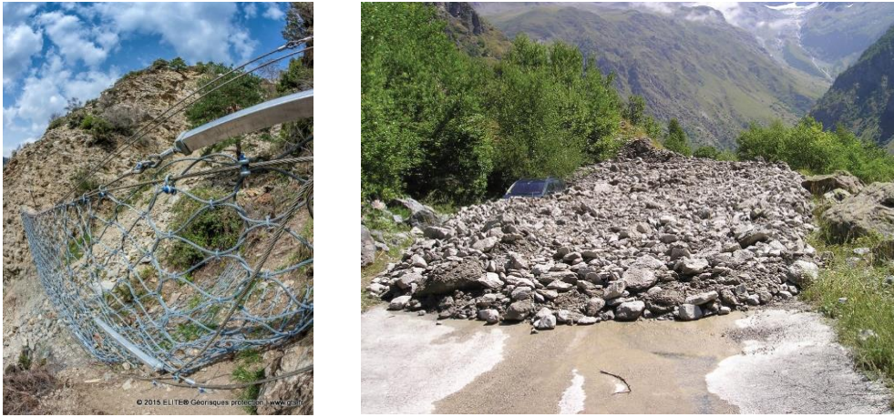
Figure 1: example of debris flow flexible fence and coarse debris flow
