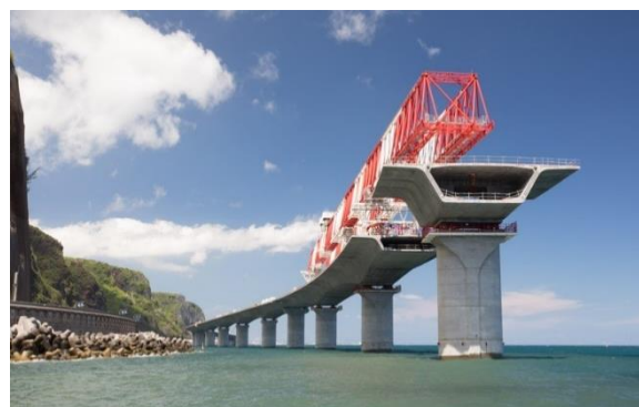
Figure 3: Viaduct under construction in 201
