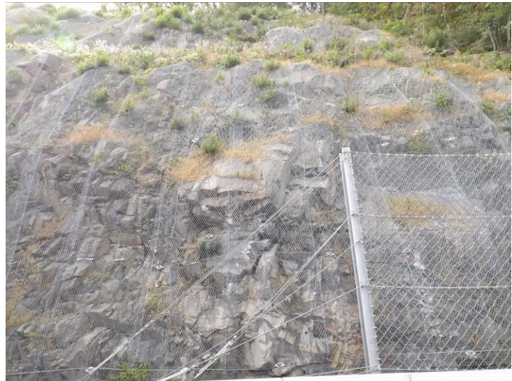
Figure 1: High-strength steel wire mesh can replace rockfall barriers with a smaller environmental and visual impact. It also requires less maintenance.
