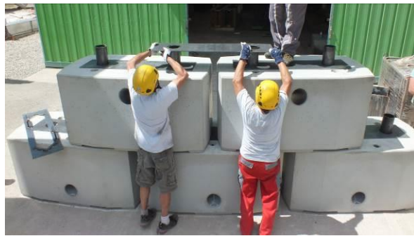
Figure 3: Bloc Armé® : Concrete blocks linked with metallic reinforcements
