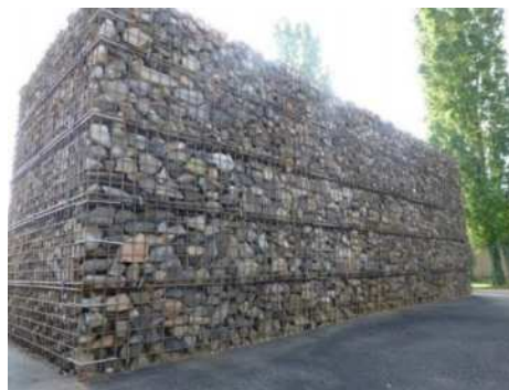
Figure 1 :Reinforced Erath protective bund
