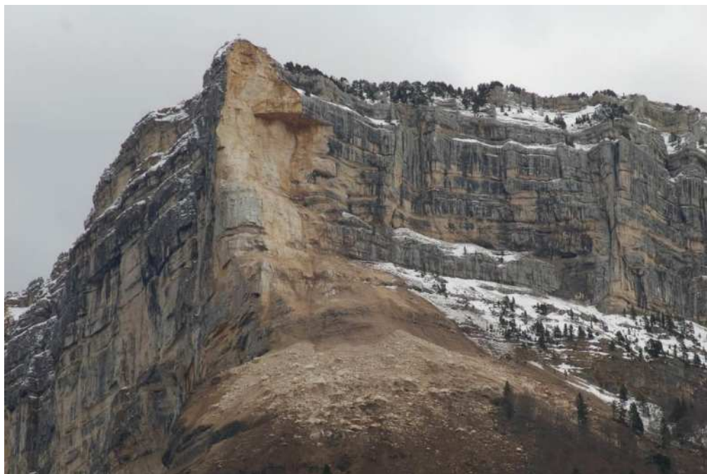
Figure 1: The NW pillar of the Mont Granier after the event
