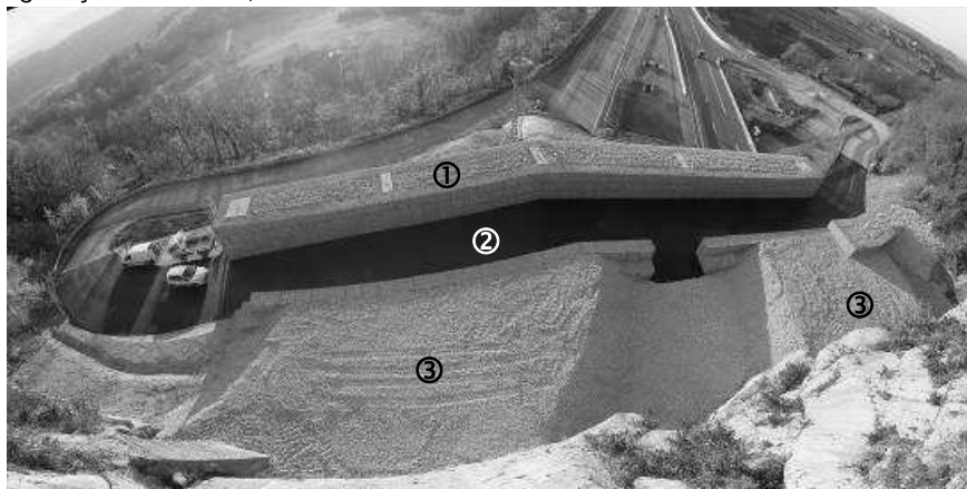
Figure 6: Sights of the finished embankment
