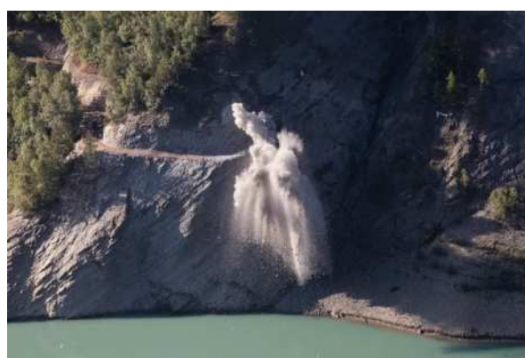
Figure 4: Mining of the central spur on the left bank
