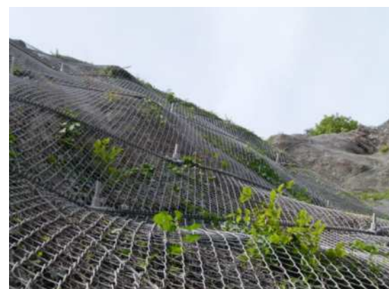
Figure 2: Unidirectional configuration - Reinforced system
