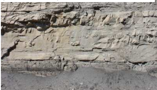
Figure 2: Application: highwall with a potential unstable block
