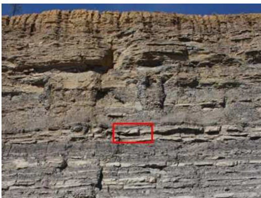
Figure 2: Application: highwall with a potential unstable block
