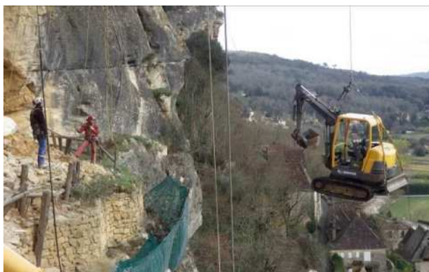
Installation of a material ropeway for removal of debris and supply
