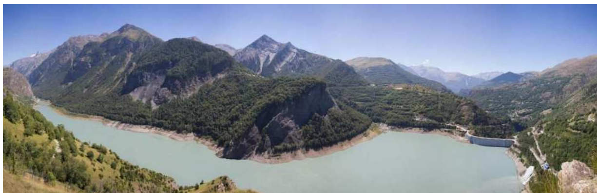
Figure 3: General view of the left bank before work
