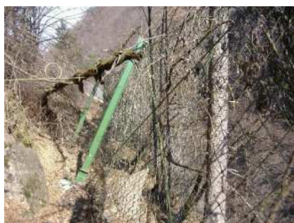
Figure 1: Flexible barrier within the PAB
