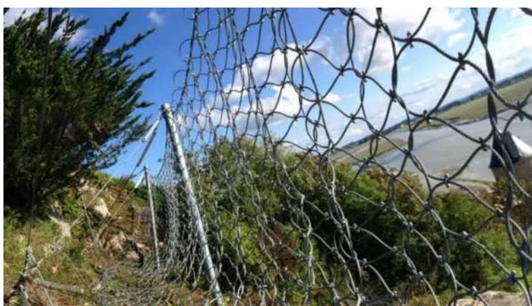
Figure 3 and 4 : Rockfall fence installed on a difficult slope and its integration with limited impacts
