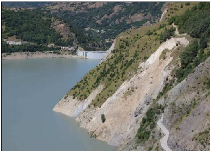
Figure 1: The slide on the right bank of the Chambon Lake.
