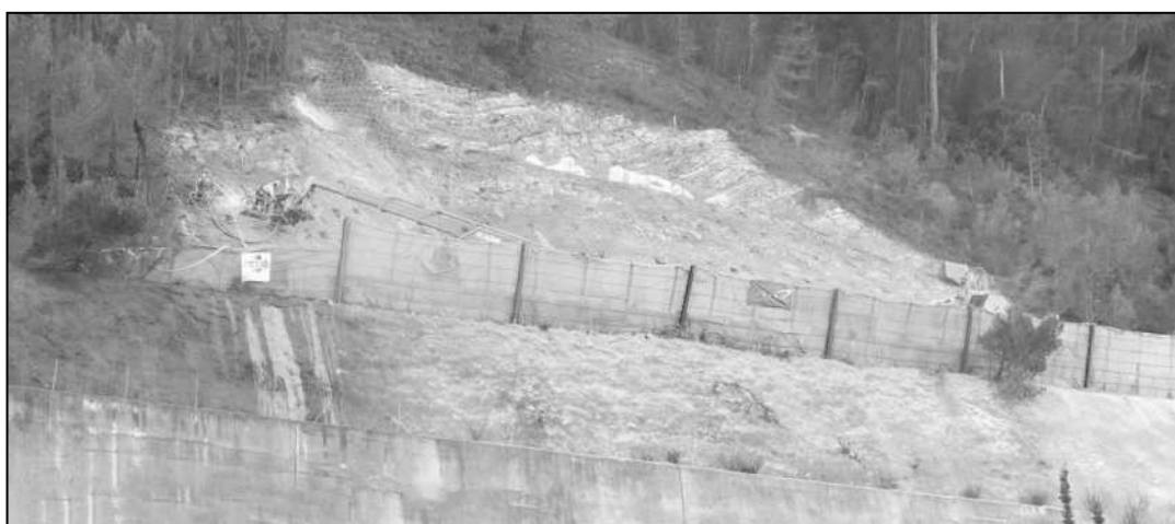
Figure 2: Works under progress
